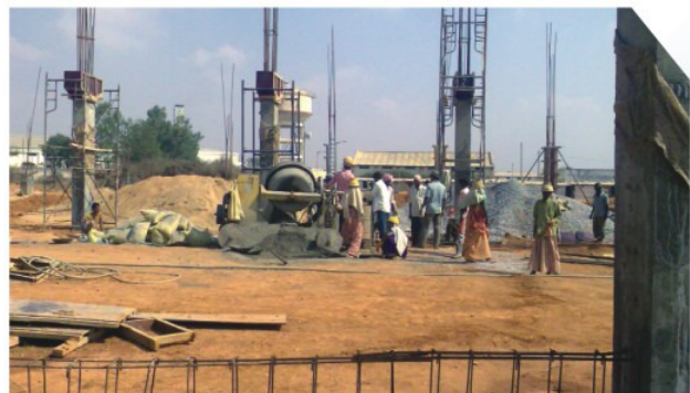
Site under Construction
